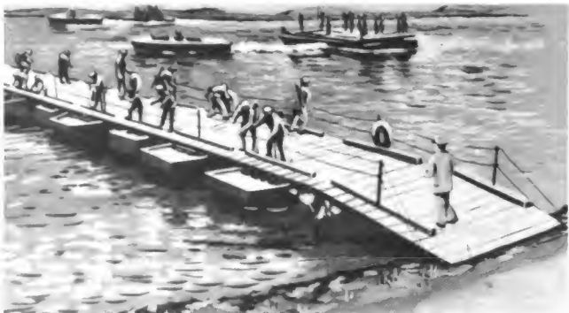
Figure 6-49. Ponton bridges. Light and heavy-weight ponton bridges are employed by the Soviet Ground Forces. The LPP light ponton bridge (above) can carry up to 40 tons, and the heavy TPP (below) carries up to 70 tons. Each ponton is carried on a single truck.
